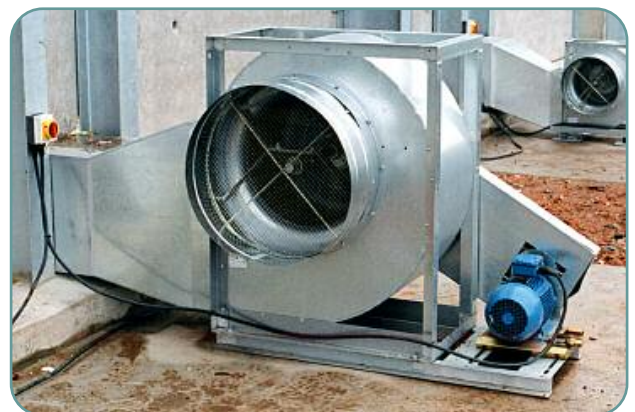
Below: Single inlet galvanised Belt Driven Centrifugal Fansets providing aeration and conditioning to a 2000 tonne flat store.
