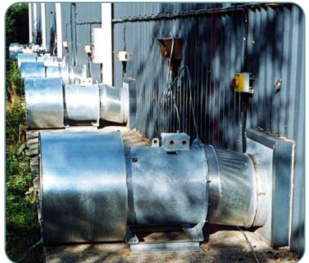
Above: 2x stage Axial Fansets and Silencers used for aeration and conditioning of a 12000 tonne oilseed flat store.
