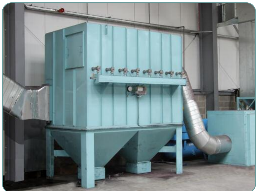
Reverse Jet Filter installed externally to the building, rated for 9750 M 3 /hr of air contaminated with grain dust, showing a Ø150mm pneumatic transfer blow-line moving the filtered dust to an elevated silo.
