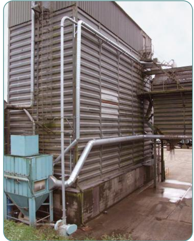
Reverse Jet Filter installed externally to the building, rated for 9750 M 3 /hr of air contaminated with grain dust, showing a Ø150mm pneumatic transfer blow-line moving the filtered dust to an elevated silo.
