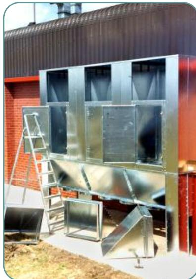
**Filter/Collector type Single Modulex:** A six bag Filter/Collection unit under construction on site. This "Modulex" concept can be delivered in flat pack for local assembly which can be convenient where access is limited and when the units are installed indoors. Alternatively, they can be delivered assembled and lifted into position with a fork lift or crane, depending on site conditions.
