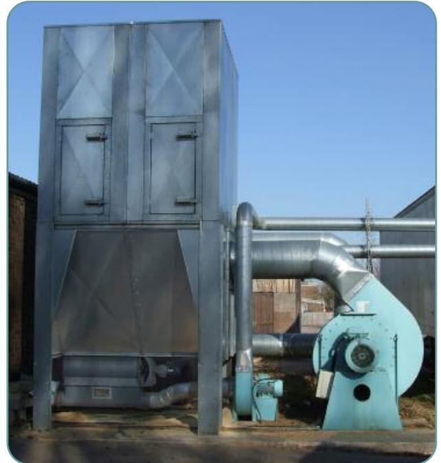
**Filter type Double Modulex:** An outdoor filter installation with a 30kW extraction fan set rated for 17000M<sup>3</sup>/hr, handling large quantities of softwood waste. This filter is fitted with a rotary valve discharge into a pneumatic transfer blow-line to transfer the waste into a sealed container for final disposal, alongside the filter.
